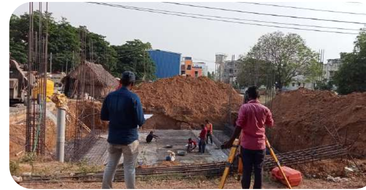
Site Marking & Excavation
