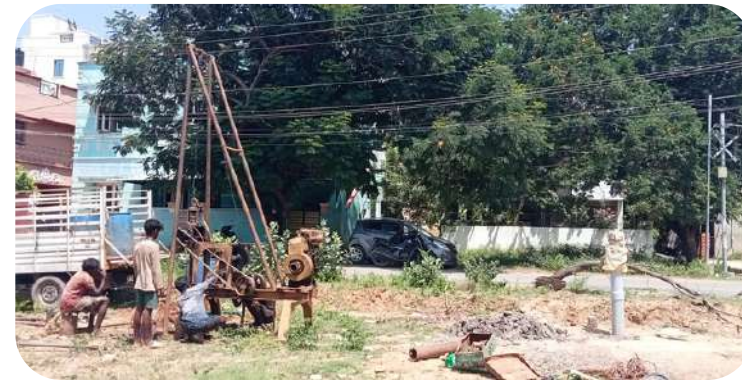
Soil Test & Structural Design
